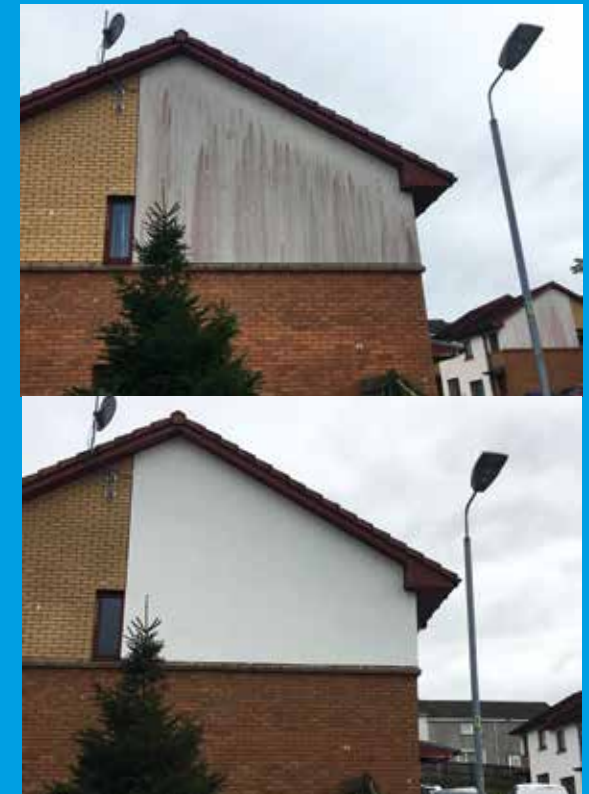
Braehead gable ends 'before and after' painter works
